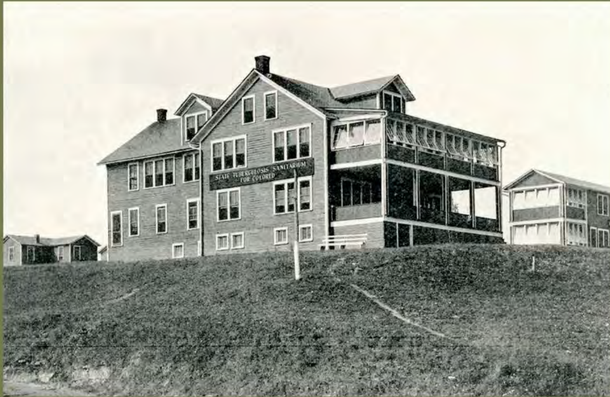
West Virginia Colored Tuberculosis Sanitarium prior to the 1939 hospital. Note the large awning windows of the "solariums" on the second floor porch and adjacent building. Patients would lie at bed rest there breathing the fresh air for several hours per day. Photo: West Virginia and Regional History Collection, West Virginia University Libraries.
