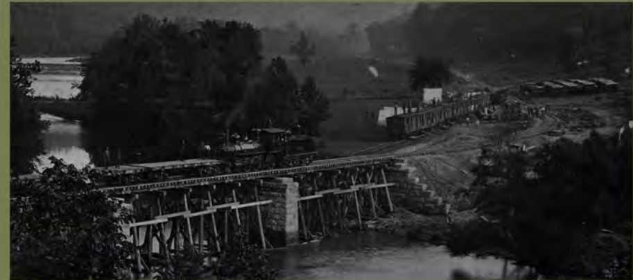
Temporary bridge over Spring Creek looking downstream on the Greenbrier soon after the track was completed to this point in 1900. Note the construction train on the bridge and, on a temporary siding, the string of camp cars which housed the construction crews. Photo: Pocahontas County Historical Society.
