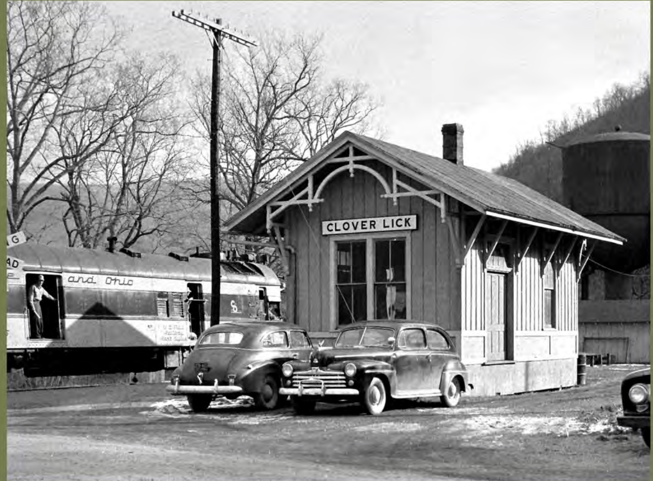
The depot in the mid 1950's. Note the water tank for steam locomotives (background right) adjacent to the depot at its former location 150 feet south of present site. Seen here also is a self-propelled railcar (no separate locomotive) that carried passengers and freight, nicknamed a "doodlebug," that came into use to save costs as railroad traffic declined. Photo: Jack and Barbara Coyner Collection.
