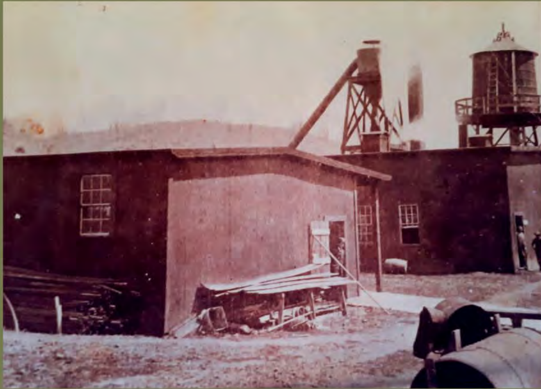
A steam engine-powered machining building and dry kiln/storage building were used to prepare and season the oak lumber for rail shipment. Photo: Glen & Twyla Diehl Collection.
