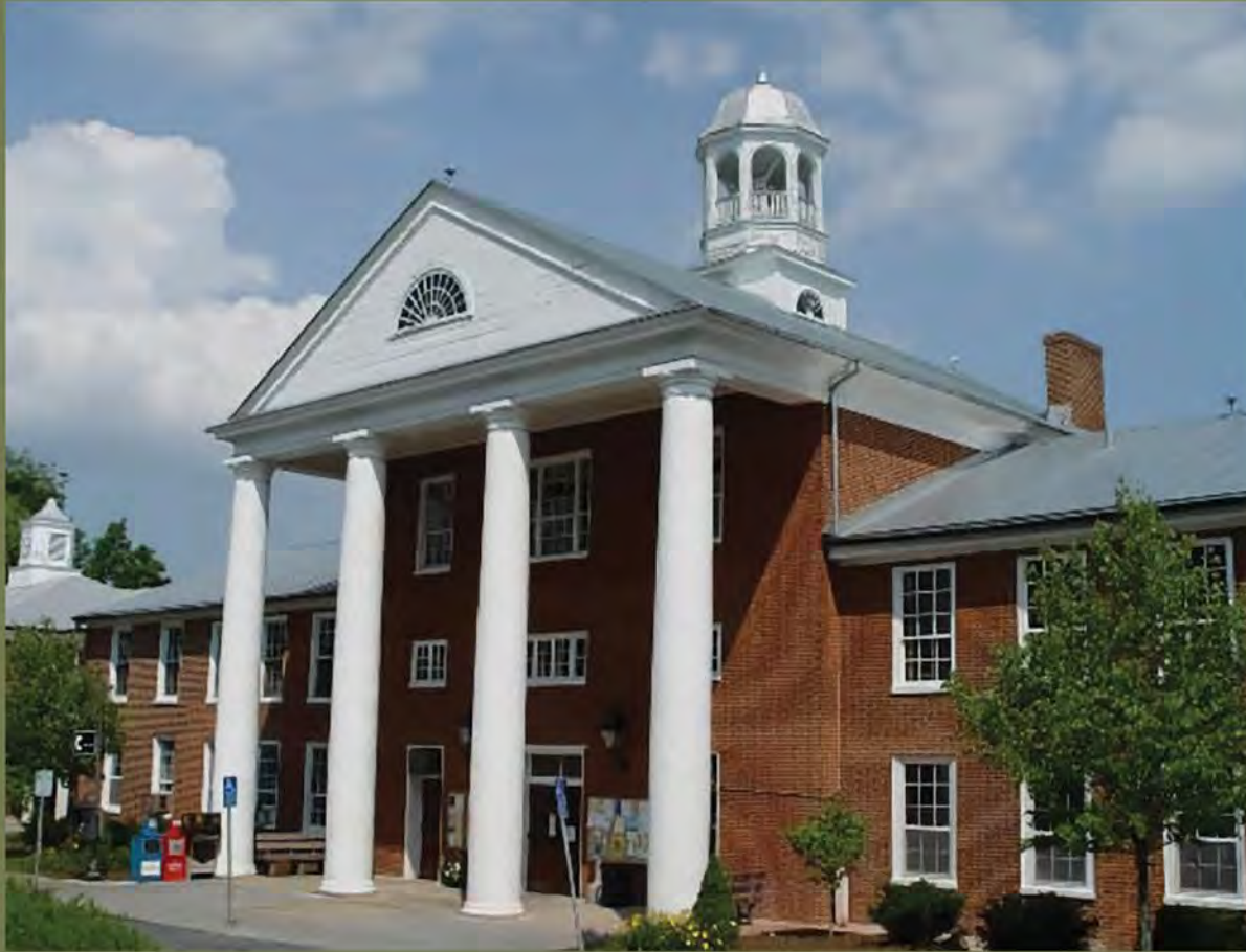
Greenbrier County Courthouse in Lewisburg
