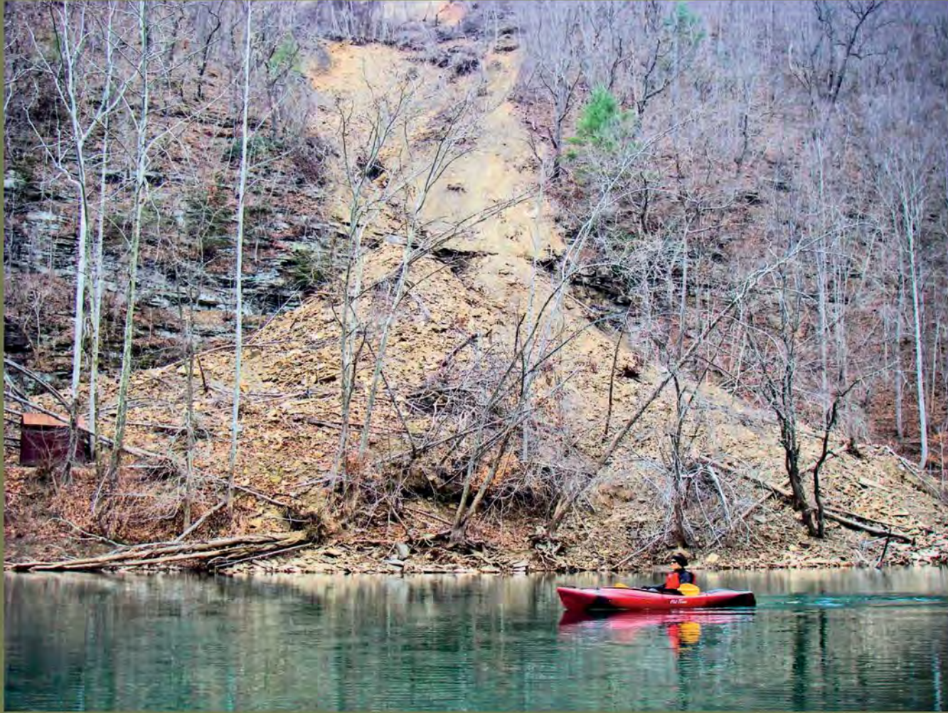
The 2016 landslide created a blockage on the Trail 400-feet long and over 100-feet high. Photo: Jack O'Connell.
